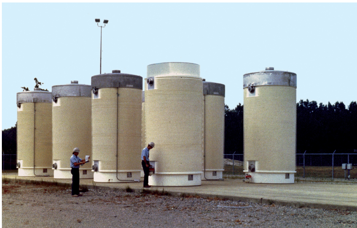
Workers, evaluating temperature readings on the outside of dry waste casks. Workers do not need to wear any protective clothing since radiation levels are negligible.
